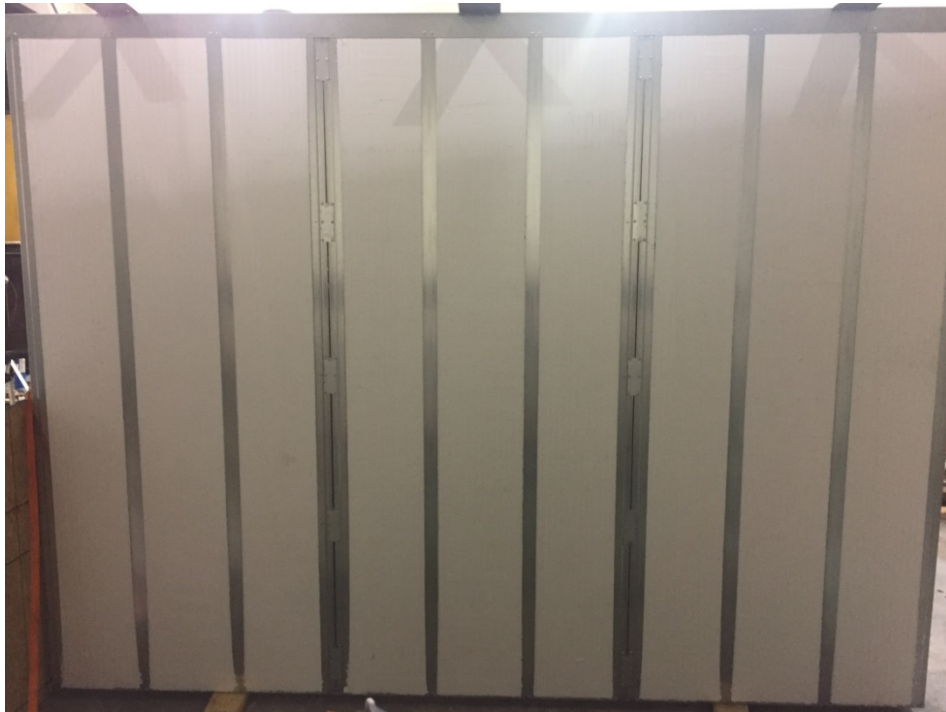
Figure 6: The unexposed face prior to the exterior gypsum board being mounted.
