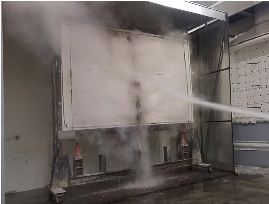
Figure 10: The exposed face at the beginning of the hose stream test.
