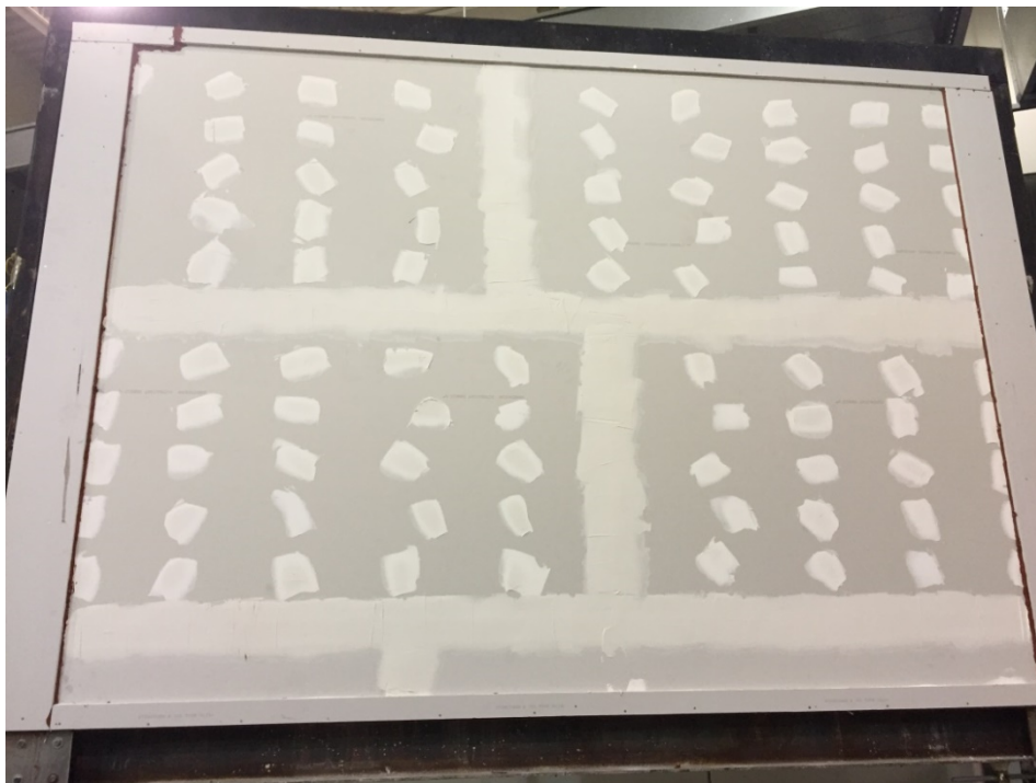
Figure 6: The exposed face prior to the fire test.
